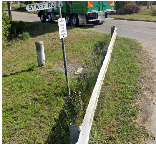
Figure 13 - Telstra Pit Staff Road & Maldon Bridge Road (Google street maps 29/07/2020)
